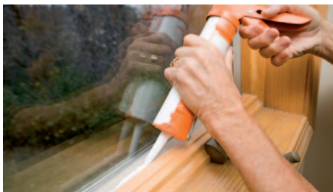
Figure 22 Application of a filled silicone window sealant
